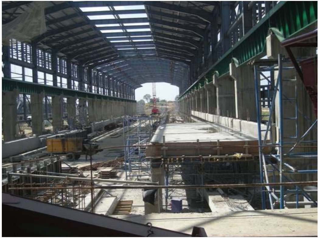
359ktpa smelter pot line - civil work nearly completed
